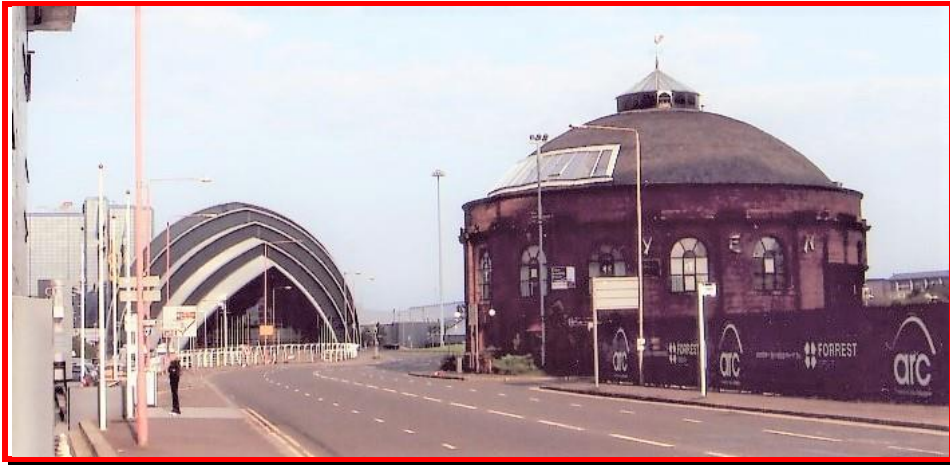
The Rotunda of the old pedestrian tunnel as it looks today
