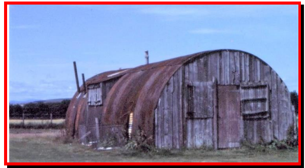
The Nissen hut just prior to demolition
