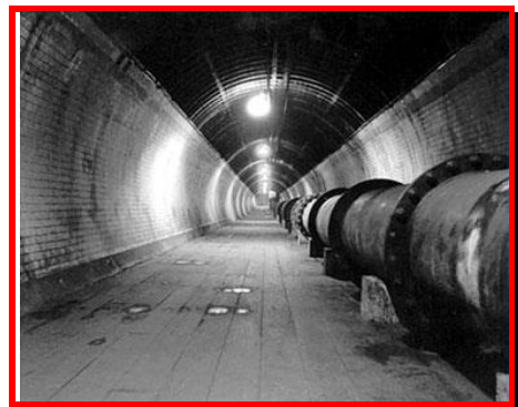
Interior of the old pedestrian tunnel
